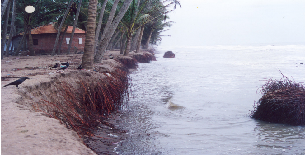
EROSION AT KAPPAKKAL BEACH (PAYYANAKKAL) AT CALICUT, KERALA
