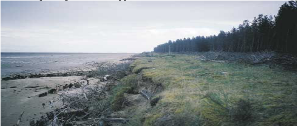
Clear felling of forestry along an eroding coastline.
