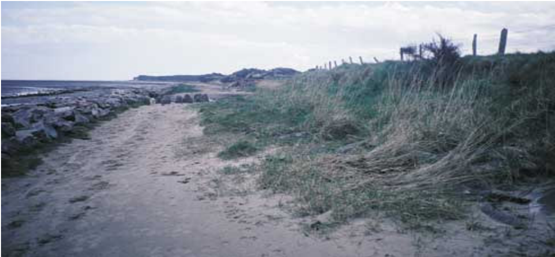
The same breakwaters as illustrated above, seven years after construction. Note relative stability of backshore.
