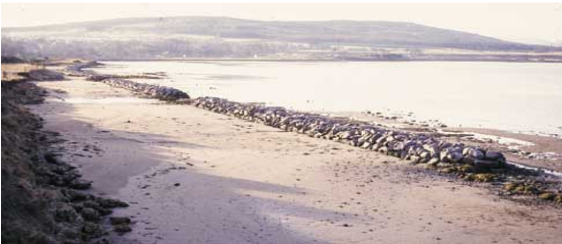
Nearshore breakwaters on the upper foreshore in the Dornoch Firth, shortly after construction.
