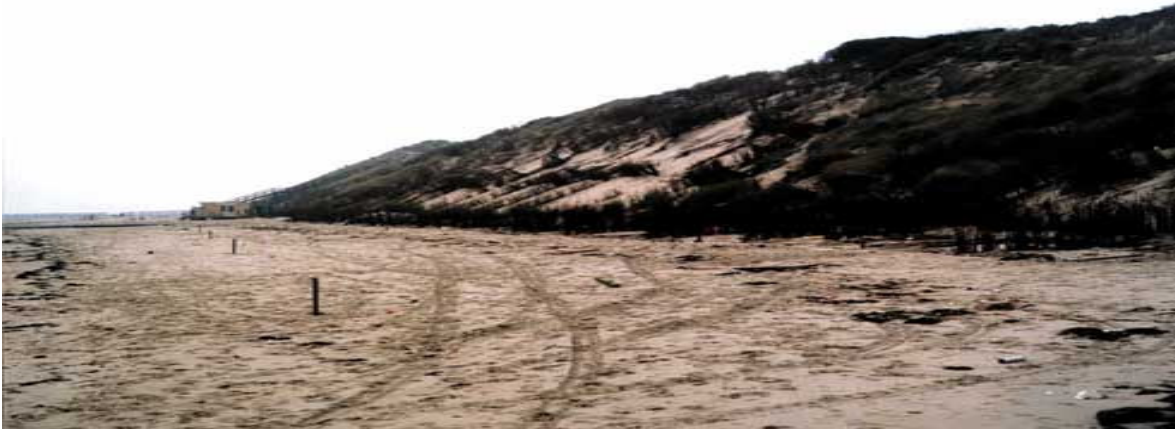
Thatching and brushwood fencing along an eroded dune face.
