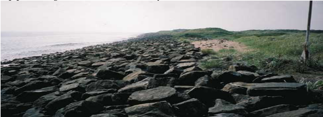
Major rock armour revetment in front of dune system.
